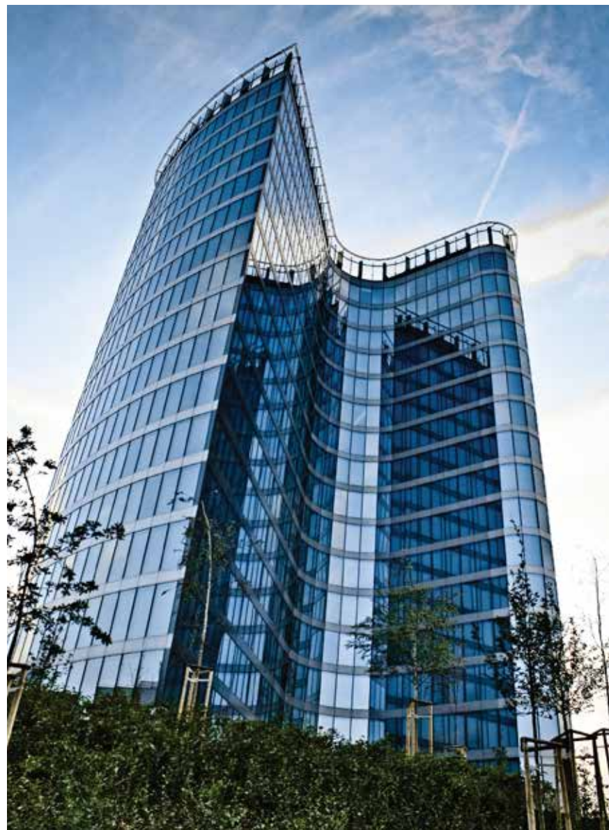
The BB Centrum in Prague rated 'good' by BREEAM
