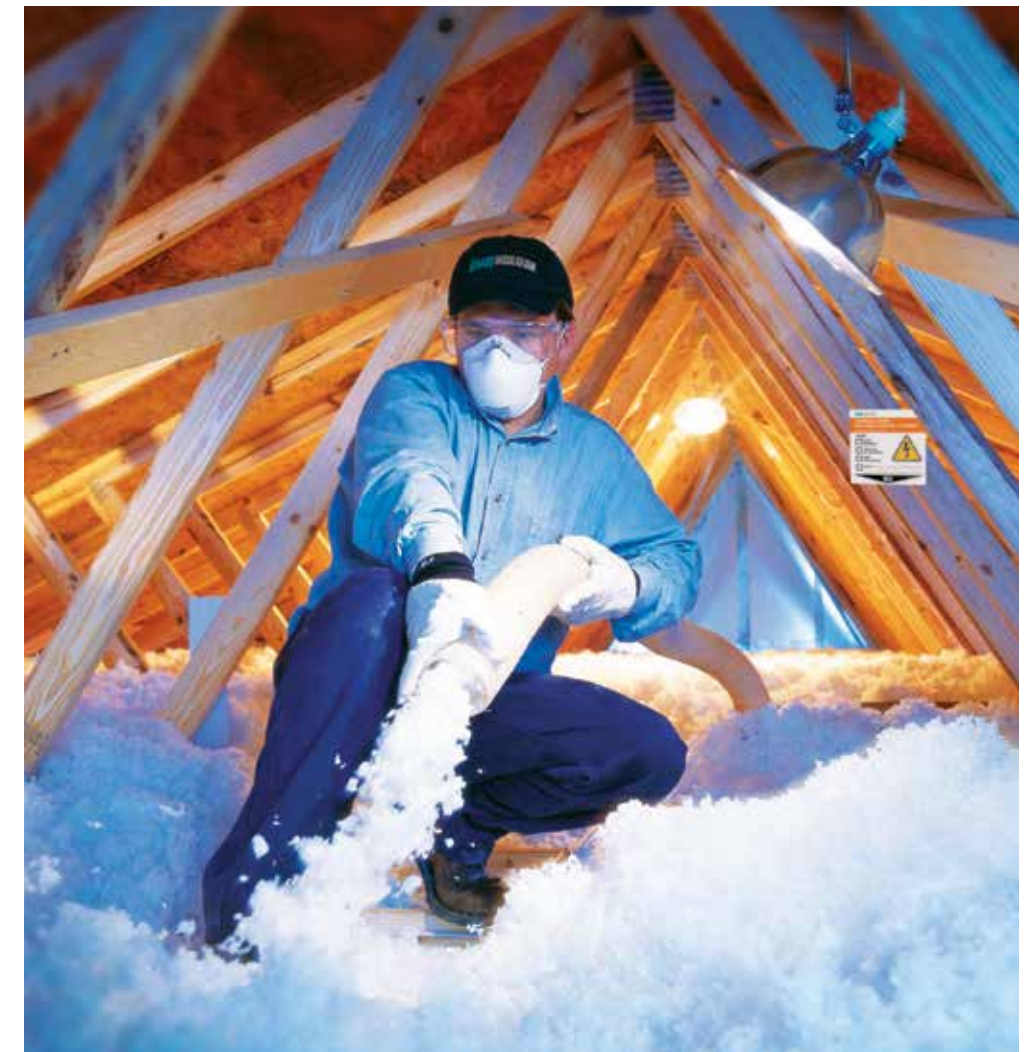
SUPAFIL can fill hard to reach loft space.
