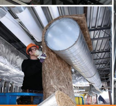
Climacoustic Duct roll is the ideal insulation for the exterior of rectangular and round sheet metal ducts, spaces and surfaces where temperature and condensation must be controlled. Climacoustic Duct roll has a premium density of 28kg/m<sup>3</sup> and a strong foil facing.
