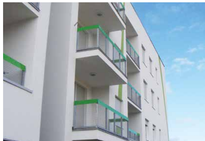
Šparna hiža', one of the first NZEB multi dwelling housing developments in Koprivnica, Croatia used Knauf Insulation Rock Mineral Wool contact facades.
