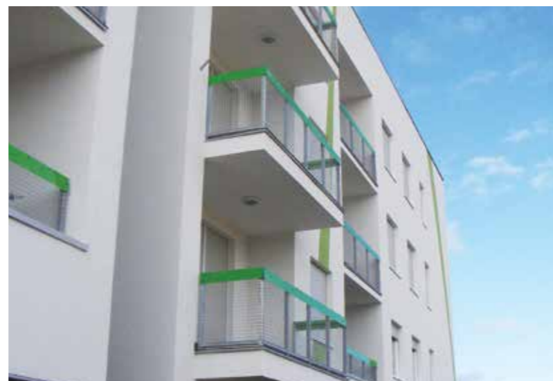
Šparna hiža', one of the first NZEB multi dwelling housing developments in Koprivnica, Croatia used Knauf Insulation Rock Mineral Wool contact facades.
